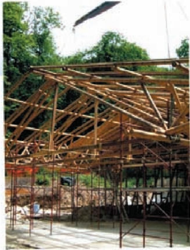
**OFX** The structure, inspired by a drawing by Colombian architect Simon Velez, who is famous around the world for his bamboo construction for the pavilion at the Expo in Hanover, consists of 15 portals positioned at intervals of 2 meters, each one supported by three pillars: one vertical and two slanting. The space between the supports of the portals is 10 meters (see the explanatory cross-sections and drawings).
